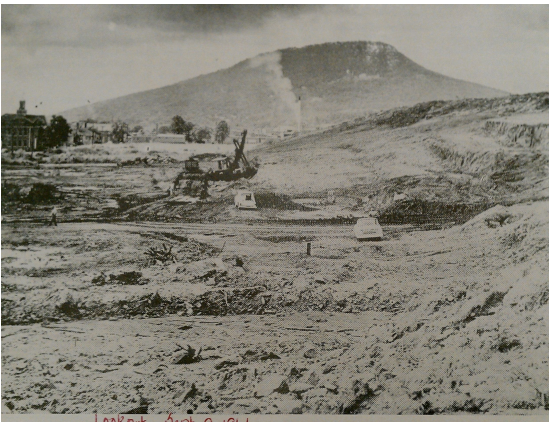
LOOKOUT, Oct. 9, 1961 NEW LOOK ON THE WEST SIDE: This shows the ground-scraping project of Urban Renewal on Chattanooga's West Side. Not a tree is left, making this photograph strangely similar to those made by Matthew Brady during the War Between the States, when the city had been stripped of trees for fuel.
